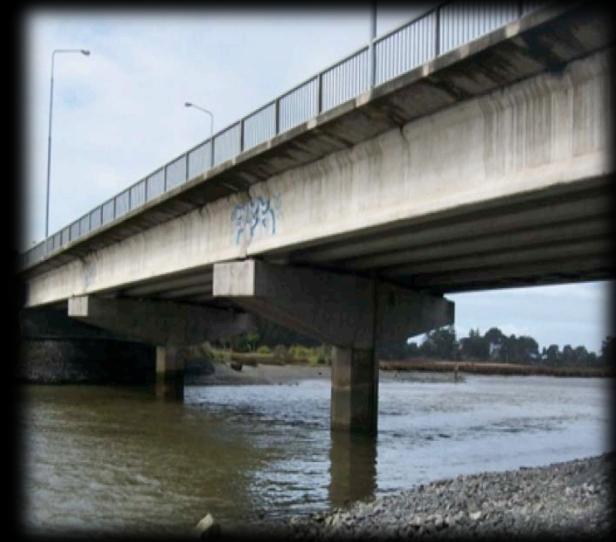
Hollow Core section (up to 22.5/25m span length)
