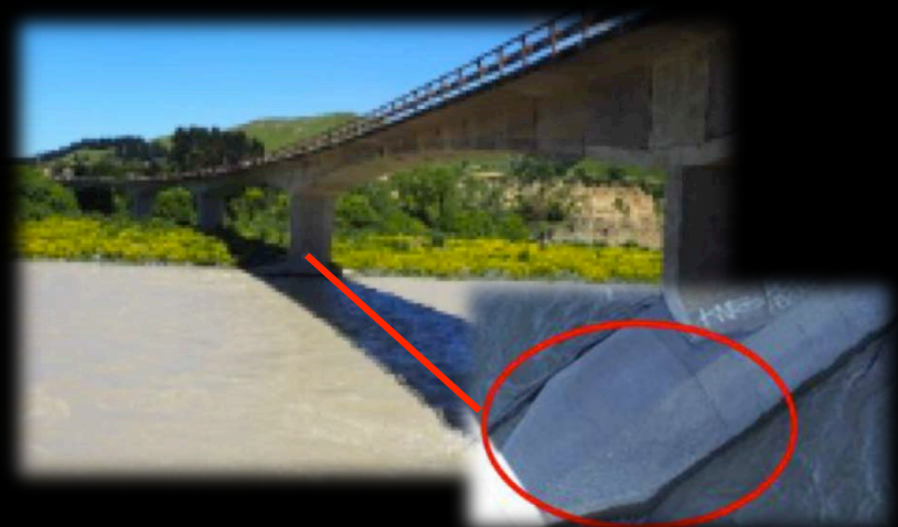
Shear cracking in the piled footing
