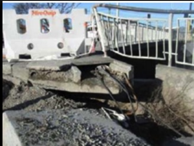
Gayhurst Road Bridge
