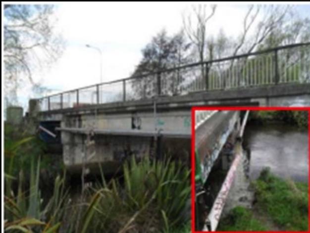
Kainga Road Bridge
