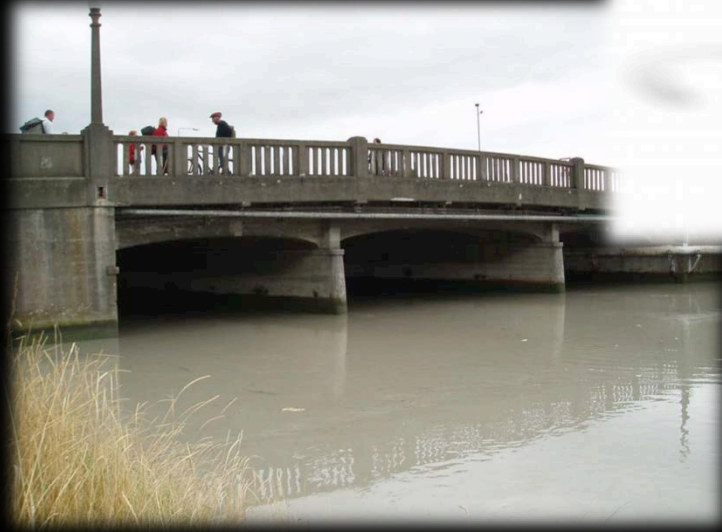
Pages Road Bridge (Integral)
