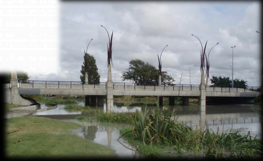
Anzac Drive Bridge (Precast)
