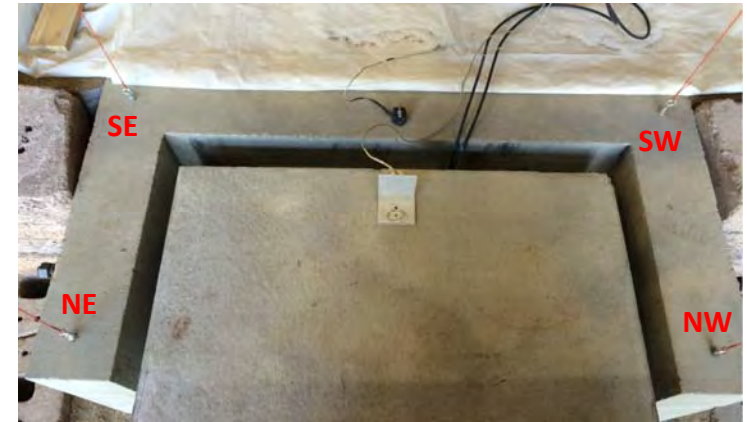
Bridge Seat Instrumentation
