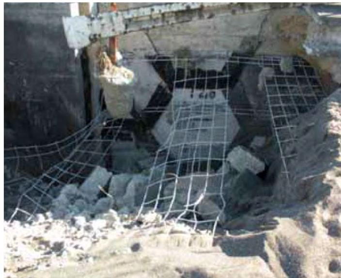
MSE wall performance in Maule Earthquake, Chile
